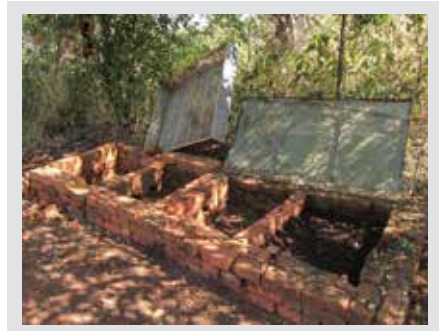
Two Tank System
