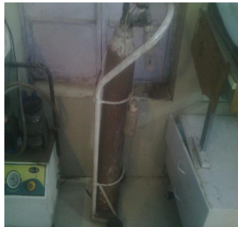
Rusted O2 Cylinder at Labor
