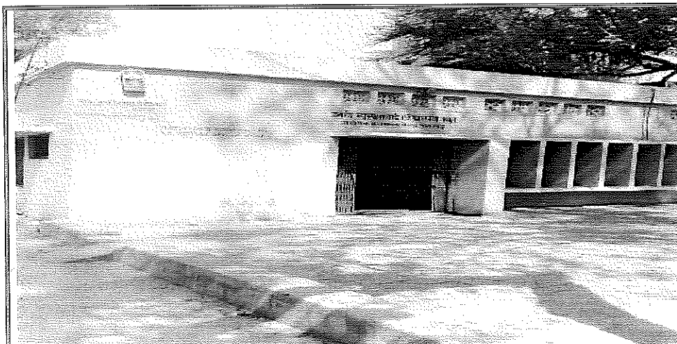
JSY Labour room, Primary Health center, Awagarh
